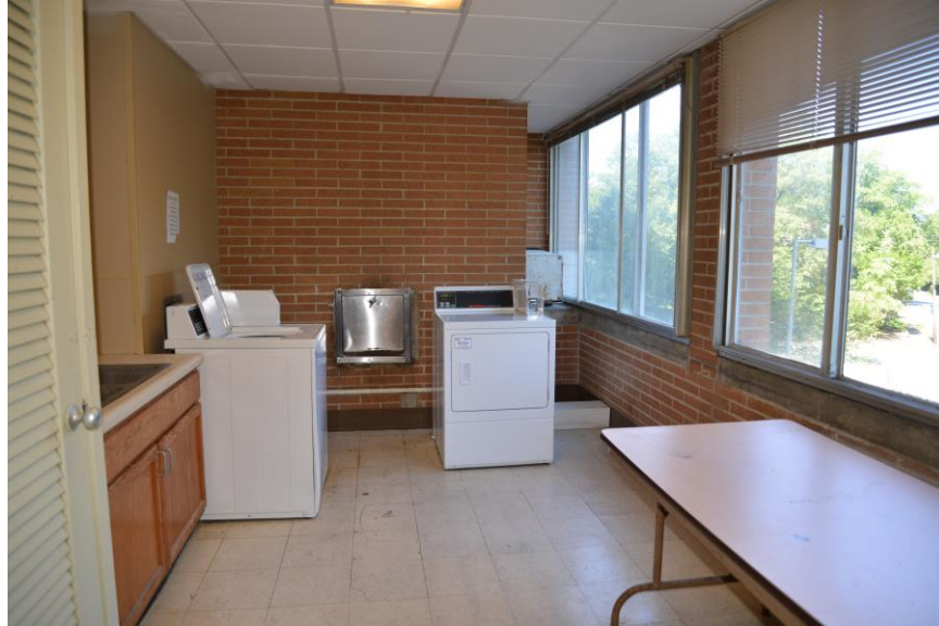
Photo 15. Interior, Second Floor, Looking West at Laundry Room, Typical
