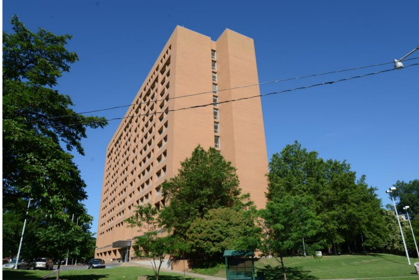
Photo 3. Exterior, South and East Elevations, Looking West
