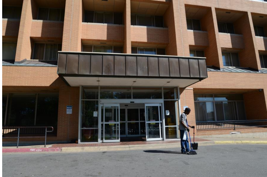
Photo 9. Exterior, South Elevation, Looking Northwest at Entrance
