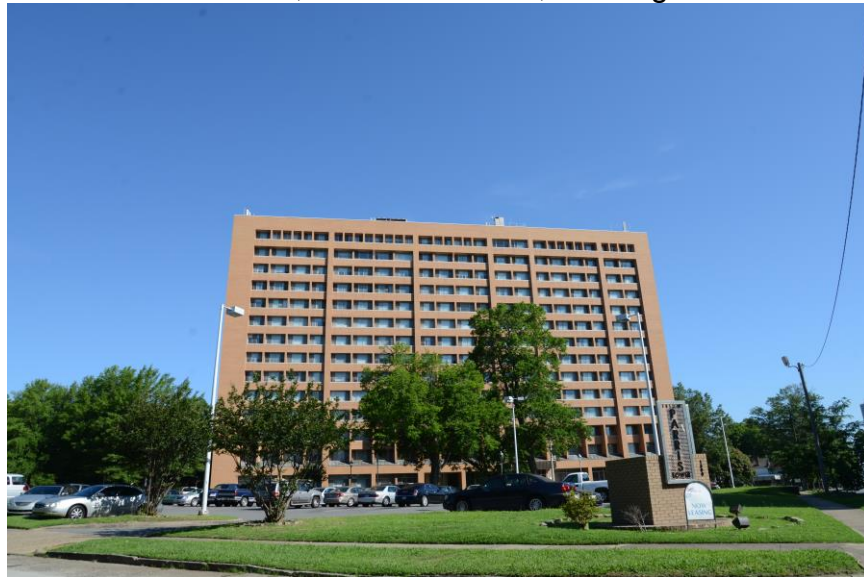
Photo 2. Exterior, South Elevation, Looking Northwest
