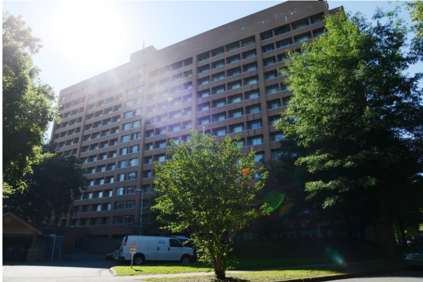
Photo 4. Exterior, North Elevation, Looking Southeast
