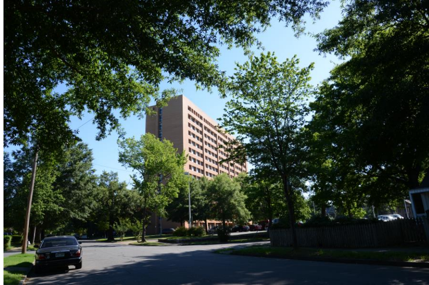
Photo 1. Exterior, South and West Elevations, Looking Northeast
