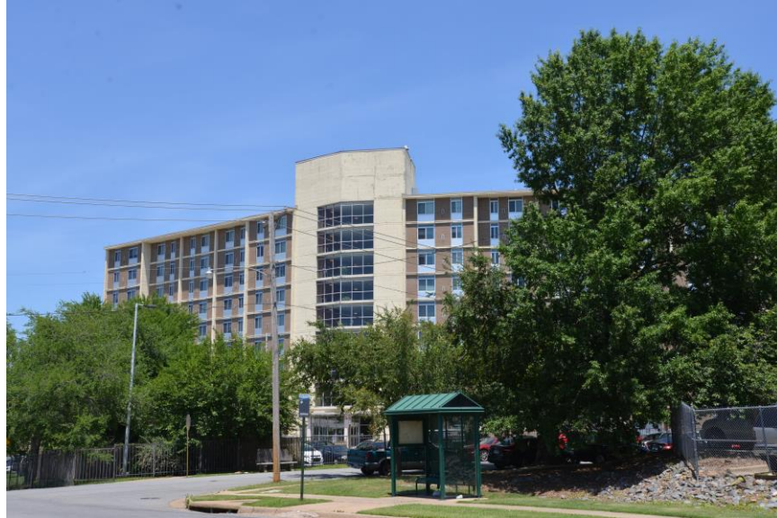
Photo 1. Exterior, West Elevation, Looking East
