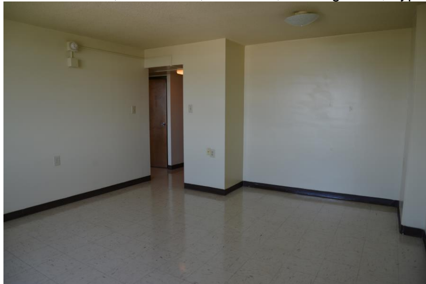
Photo 16. Interior, Ninth Floor, Unit #910, Looking West, Typical
