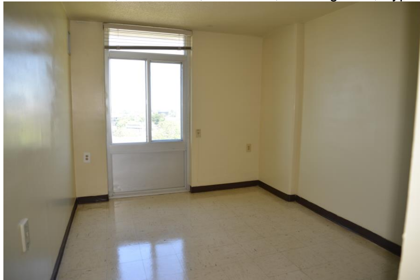
Photo 14. Interior, Ninth Floor, Unit #910, Looking East, Typical
