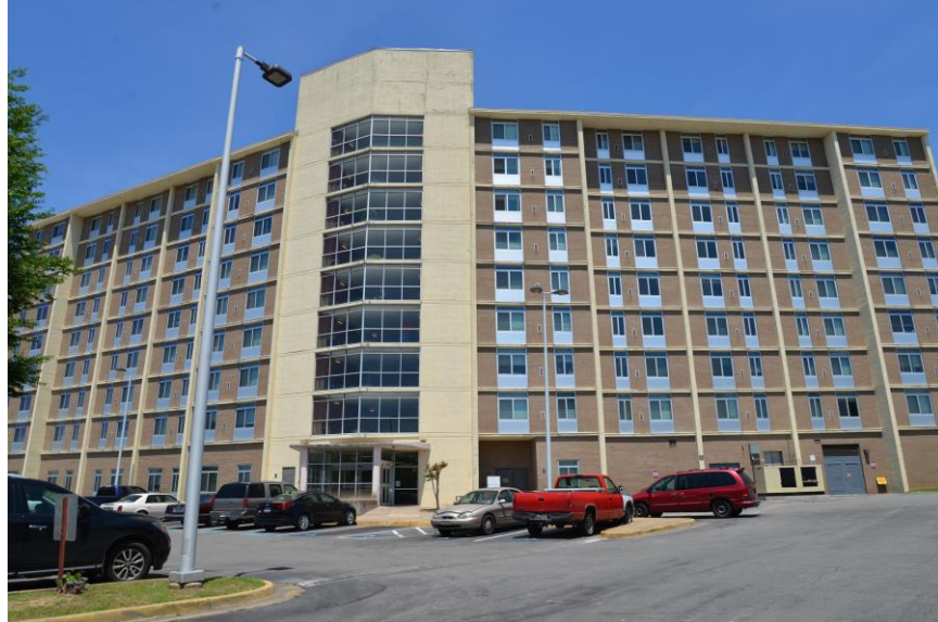
Photo 5. West Elevation, Looking East
