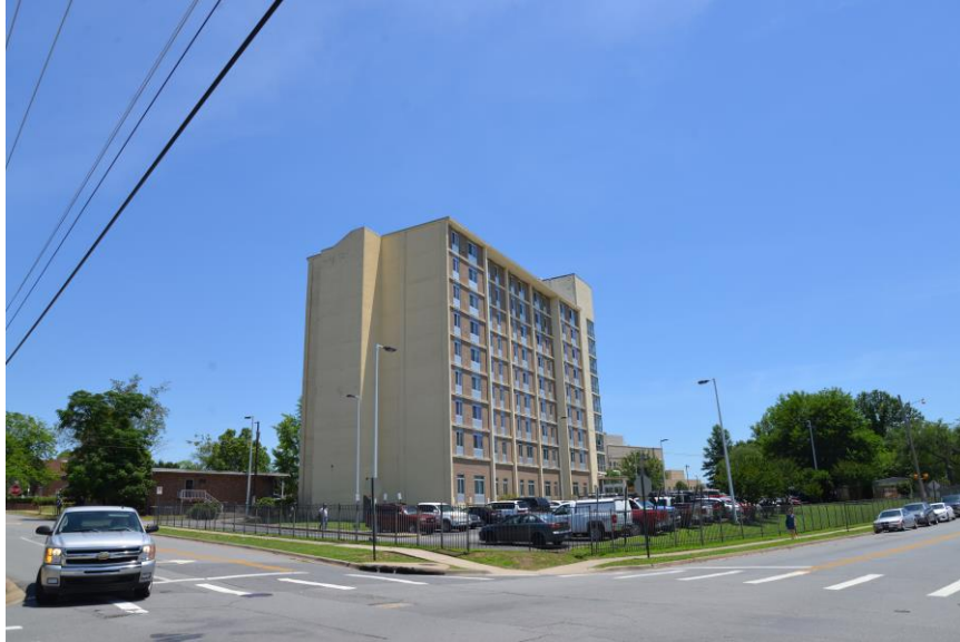
Photo 3. Exterior, West and North Elevations, Looking South
