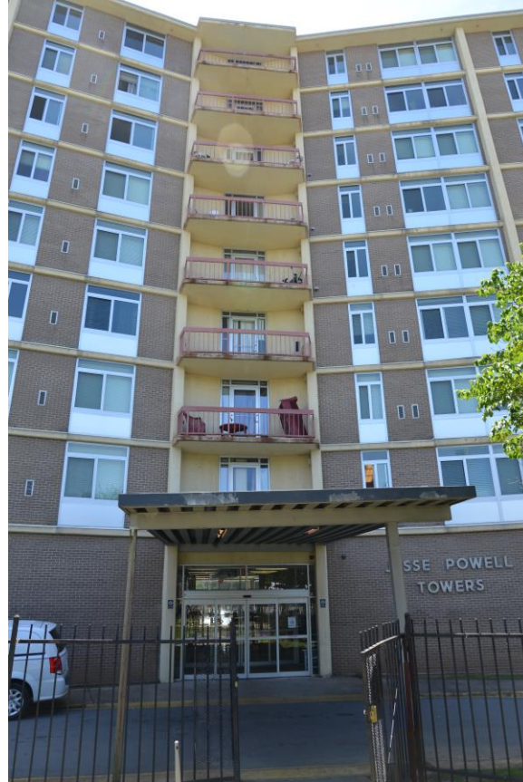
Photo 7. Exterior, East Elevations, Looking West at Entrance
